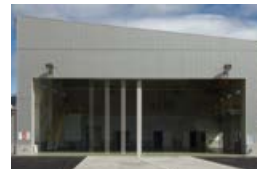
Pillar is moving
