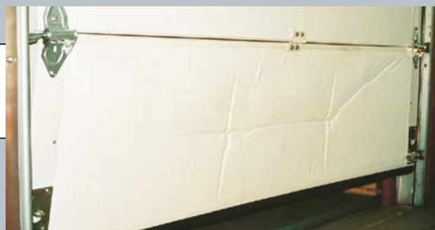
Restored (After Collision)
